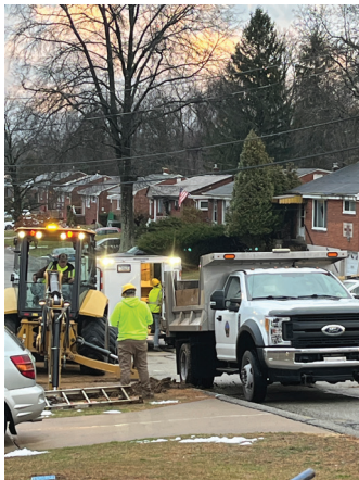
Repairing a water break on Faber
