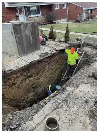
Repairing a water valve on Klementina
