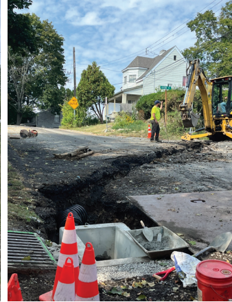
Rebuilding storm sewers on Volta
