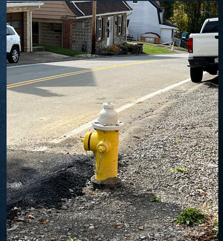
Pittview Hydrant Relocation
