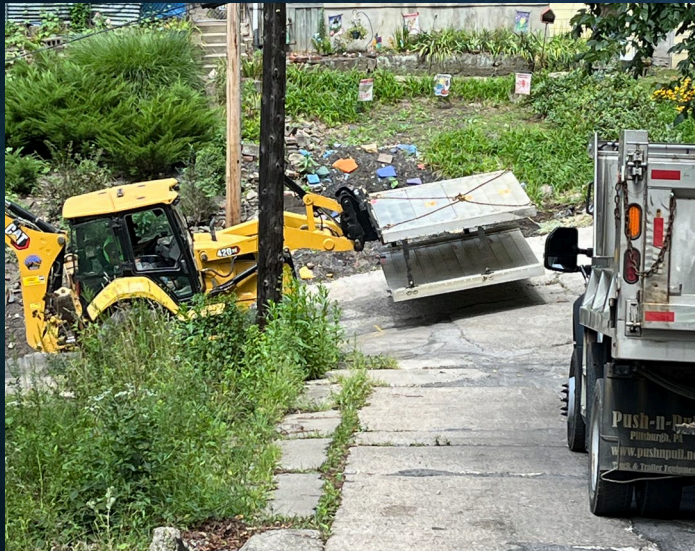
Sanitary Sewer Replacements Mauch Street
