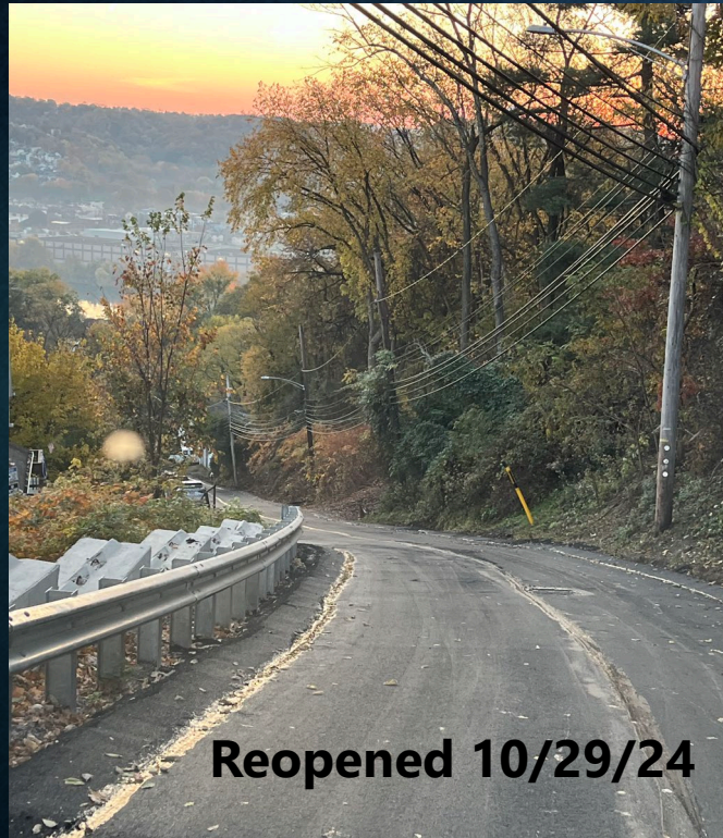
Logan Street Retaining Wall
